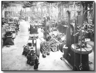
Early production, on the floor in the foreground can be seen a variety of castings ready for machining or part machined. In centre picture a couple of horizontal engine cylinder blocks. In the background at least two crankshaft lathes.
